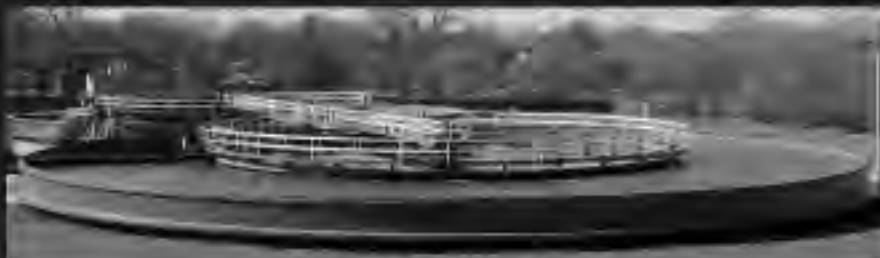
Wastewater Treatment Solutions
